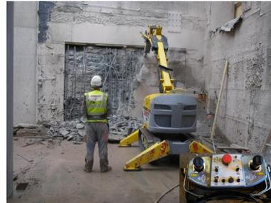
Fig. 1: An operator driving a Brokk demolition working machine. The controller interface is shown bottom right.
