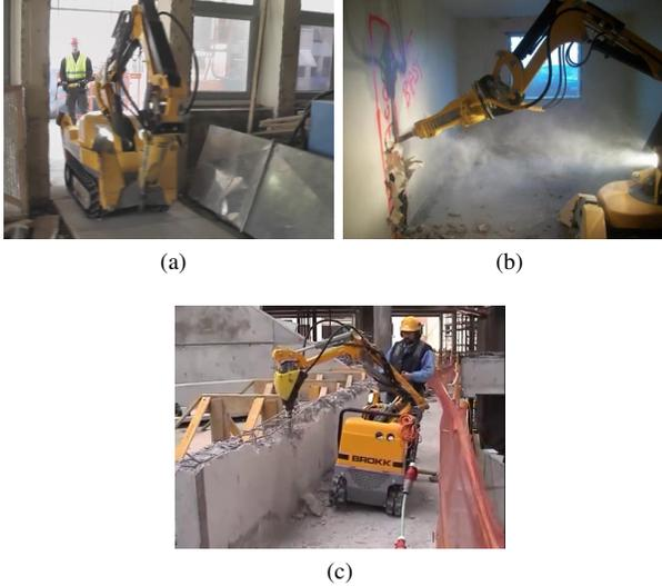
Fig. 2: Typical tasks in a demolition environment: (a) driving in narrow areas; (b) making a trace on a wall; (c) driving the demolishing arm and the mobile platform combined.
